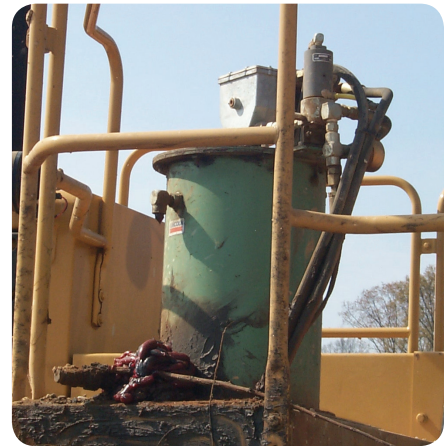
Over-filled reservoir with no overflow prevention system
